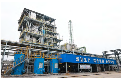
The exhaust gas treatment system enables waste heat recovery and low-emission desulfurization and denitrification of incinerated gases.
