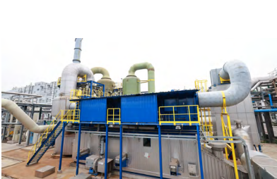
Regenerative Thermal Oxidizer (RTO) with a treatment efficiency of up to 99%.
